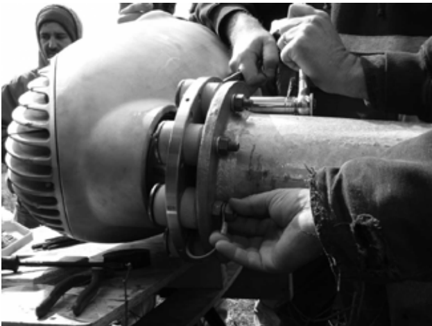
Fig. 13 Grounding turbine to tower
